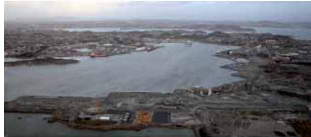
2. Foundation work for the storage tank is in progress.
