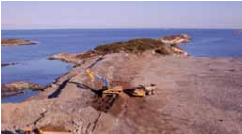
1. Start of plant construction.
