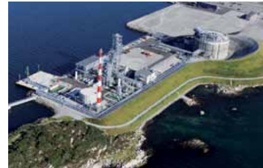
9. The plant is ready for commissioning.
