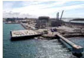
5. The quay facilities are under construction.
