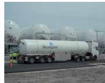
10. Øra LNG terminal was completed in the summer of 2011.
